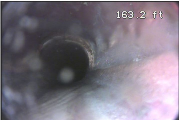
Drain waste pipe connection
