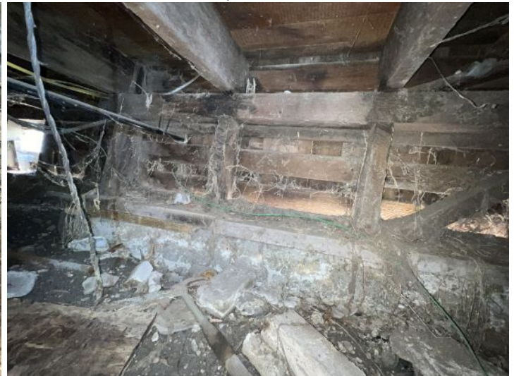
The cripple walls have been seismically displaced or have settled out of plumb, and should be evaluated by a specialist.
