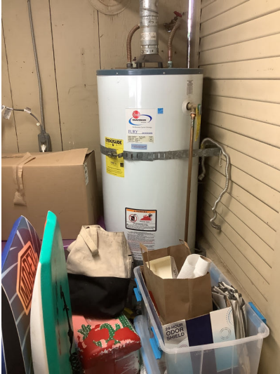
Hot water is provided by a 40 gallon gas water heater that is located in the laundry room.
