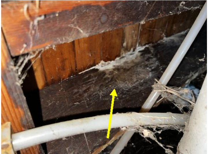
There are moisture stains beneath the bathroom which should be evaluated by the termite inspector.
