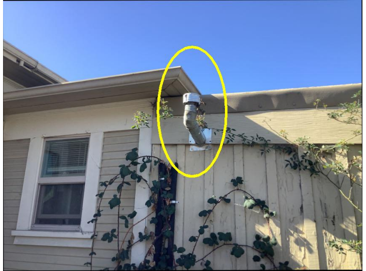
The vent pipe should extend at least 3 feet above the roof line and a minimum 5 feet above the flue collar, to safely discharge the bi-products of combustion beyond the residence, and should be serviced.
