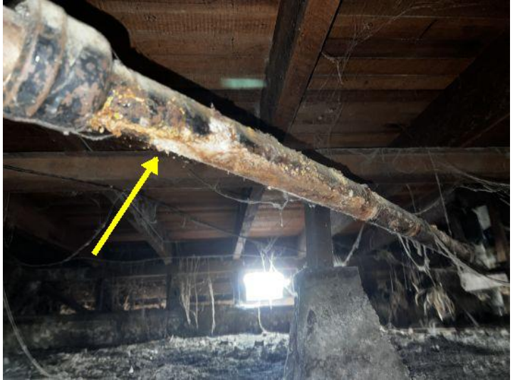
The cast iron drain waste pipes in the crawlspace are beyond their designed life, portions are rusting and should monitor for replacement.
