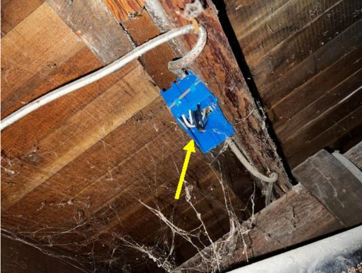
There is an open electrical junction box, which presents a fire hazard. All junction boxes should be sealed so that any arcing or sparking would be contained within the box.
