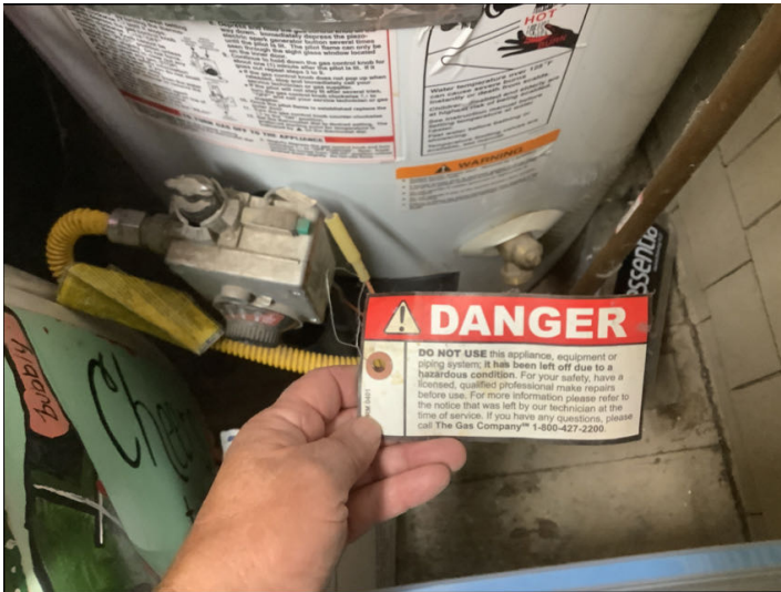
The water heater has been red-tagged by the Gas Company and should be evaluated by a licensed plumbing Contractor.
