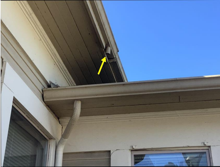
Some downspouts are missing or need to be reconnected, and should be serviced.
