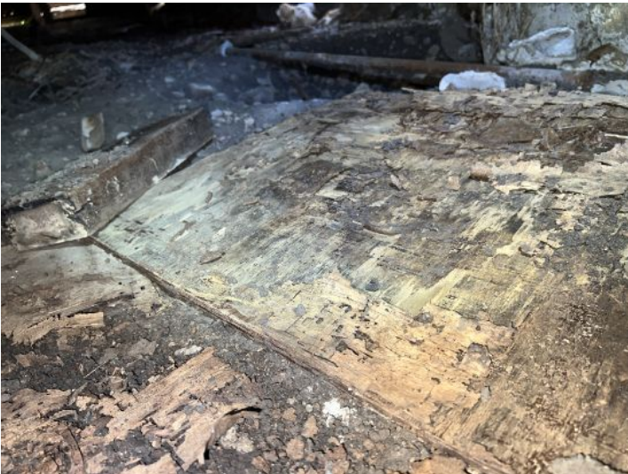
There is cellulose debris in the crawlspace that should be removed.
