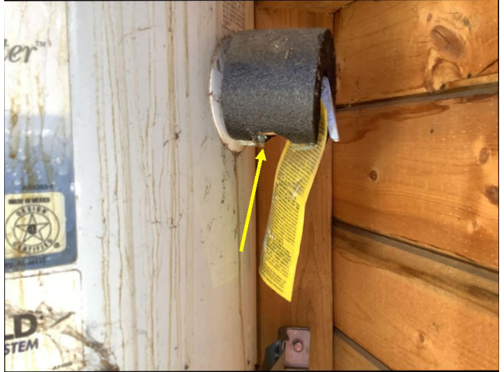
The pressure relief valve on the water heater does not have a discharge pipe. One should be installed to terminate no more than 24 inches above grade and no closer than 6 inches to it and be directed down towards the ground.
