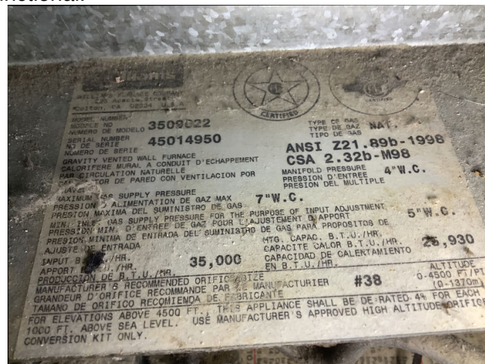
Furnace Brand--Williams Model--3509-022 Manufactured 2001
