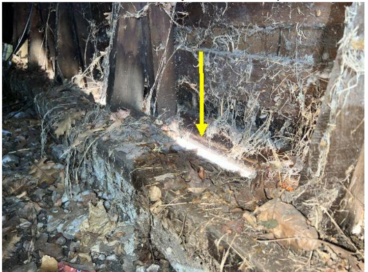
There are gaps or openings which could allow pests to enter. We recommend they be covered with 1/4 wire mesh to prevent rodent access.
