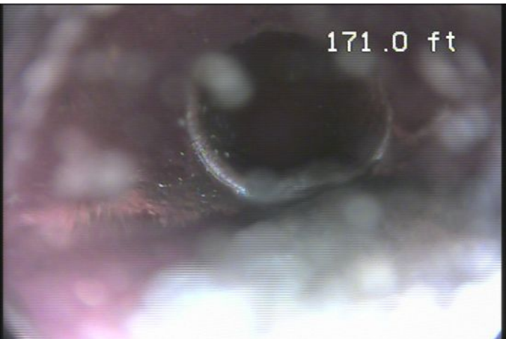
Drain waste pipe connection
