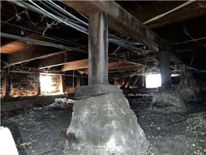
Concrete is sloughing off the foundation walls due to its age which should be evaluated by a foundation contractor.
