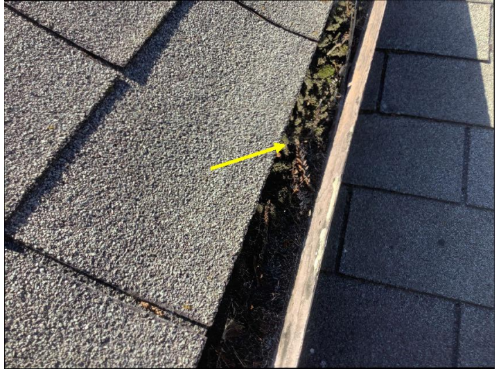
The gutters need to be cleaned to drain properly.
