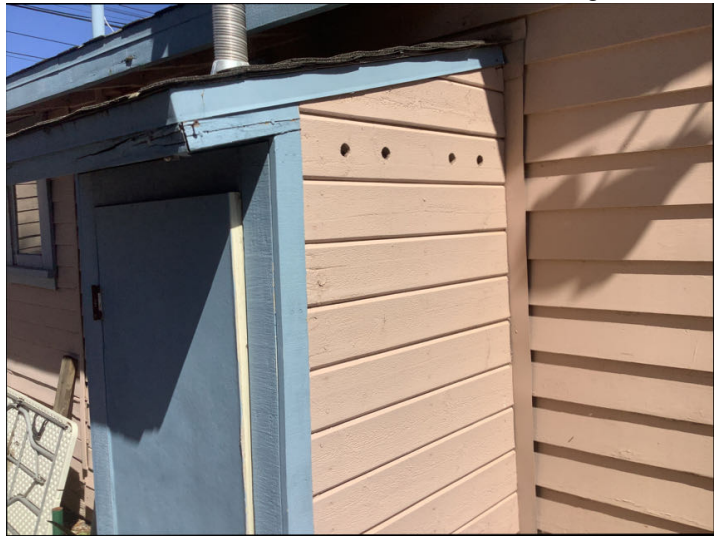
There is inadequate combustion air vent ports on the water heater door to achieve complete combustion. We recommend installing new ventilation port screens or enlarging the existing ports to current standards.
