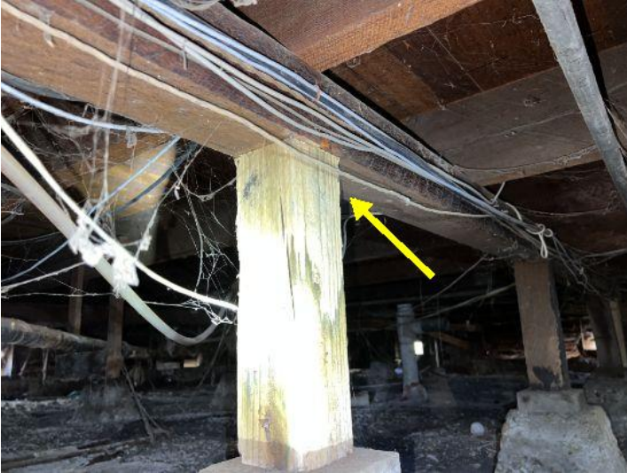
We recommend metal connectors be added as part of an upgrade to the posts and piers.
