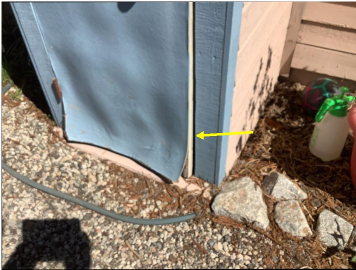
The base of the water heater closet door is moisture damaged and delaminating, and should be repaired.
