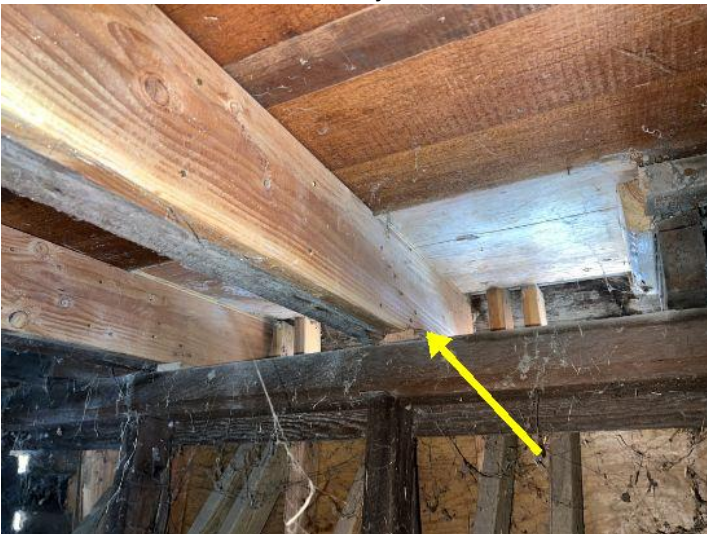
We noted repair made. The repairs appear to be a stop gap and not very effective. We recommend further evaluation by a qualified licensed foundation specialist.
